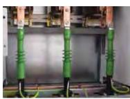
AIS20 with mechanical cable lug
